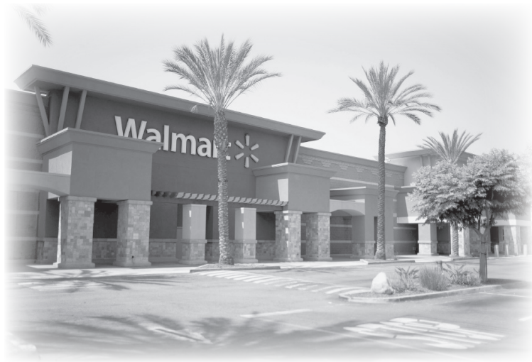
The company reopens Pico Rivera site five months after claiming to need to close to repair plumbing problems.
